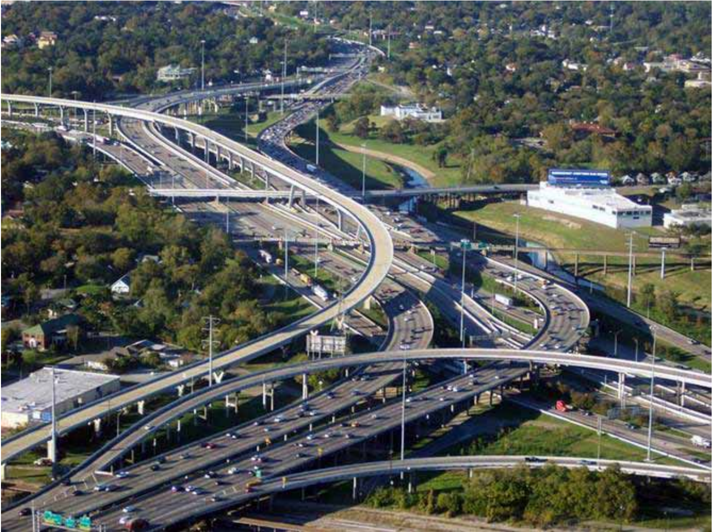
Interstate 10 Highways Interchange..... Houston , Texas
