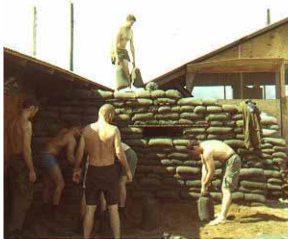
Building Solid Anchor
